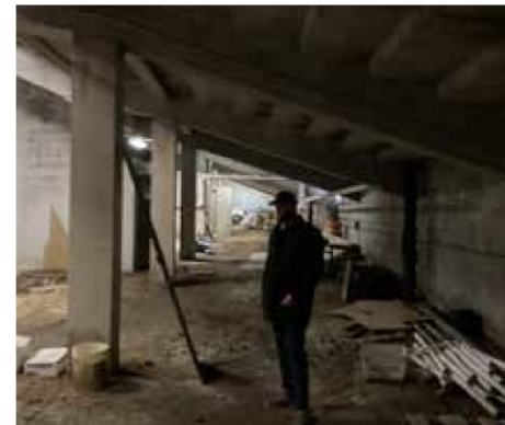
Space Under Grandstand
